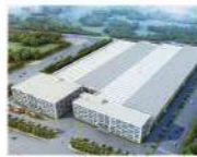
Intelligent comprehensive production base
